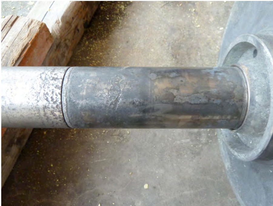
Figure 15: Corrosion on a stainless steel shaft
