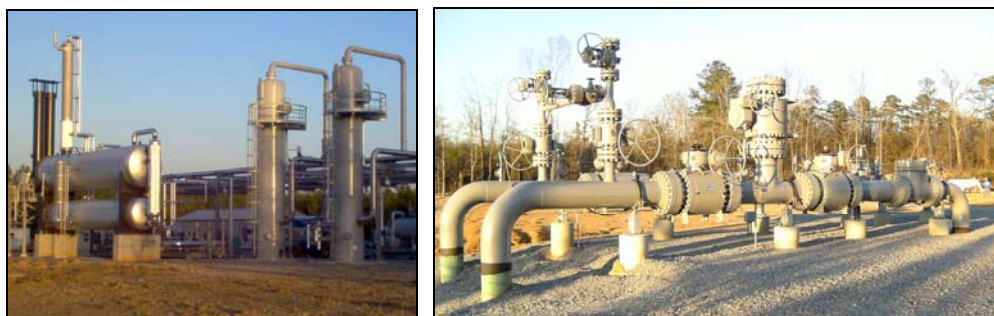
Figure 2. Example Sources of High Purity CO 2 and Low H 2 S Streams (CO 2 Dehydration Unit and CO 2 Piping)
